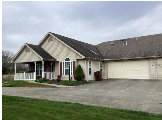
Quadraplex exterior overview
