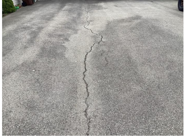
Driveway cracks
