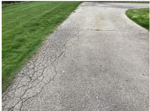
Driveway cracks
