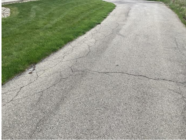
Driveway cracks
