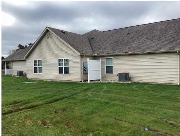
Vinyl siding overview
