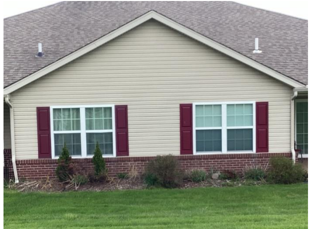
Vinyl siding overview
