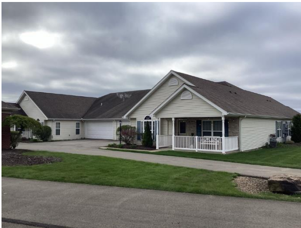
Quadraplex exterior overview
