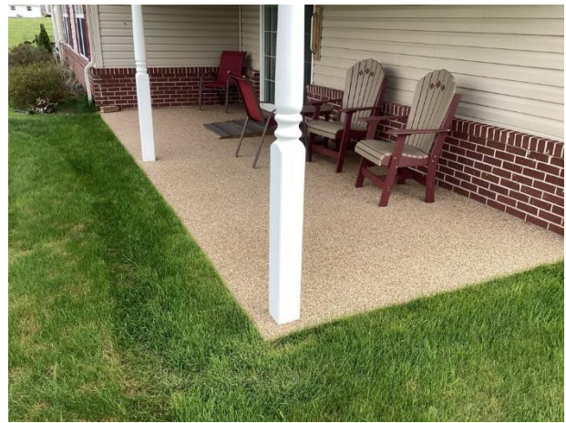
Patio in good condition
