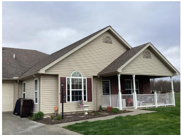
Vinyl siding overview
