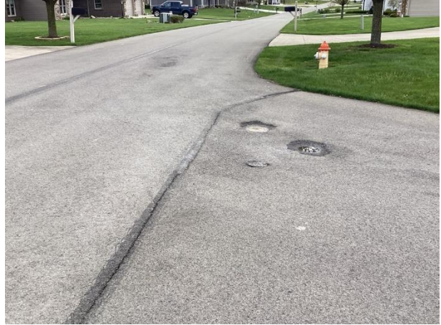
Isolated pothole
