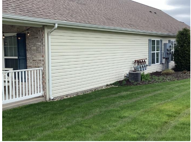
Vinyl siding overview
