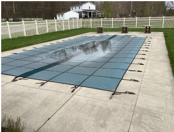
Concrete pool deck overview
