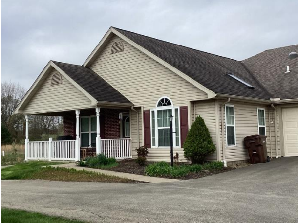
Vinyl siding overview
