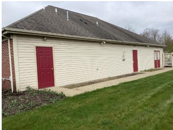
Vinyl siding overview
