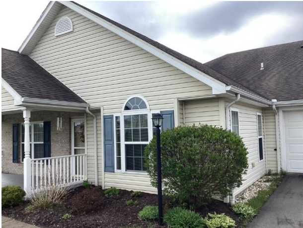
Vinyl siding overview
